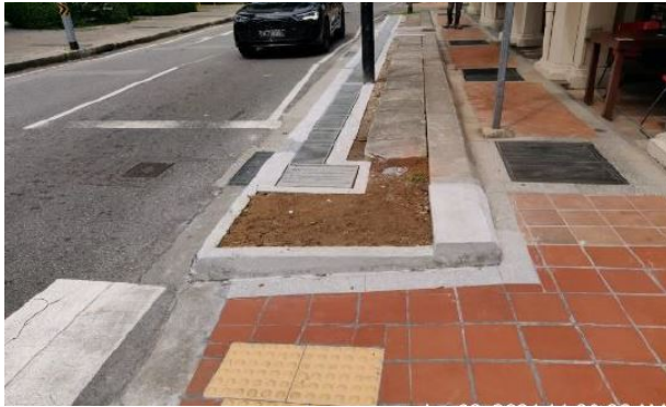
Figure 25: Retiling of the pavement
