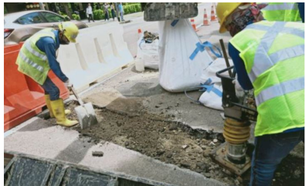
Figure 7: Backfilling the trial trenches
