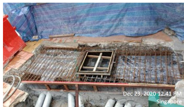
Figure 24: Laying of the Rebar slab
