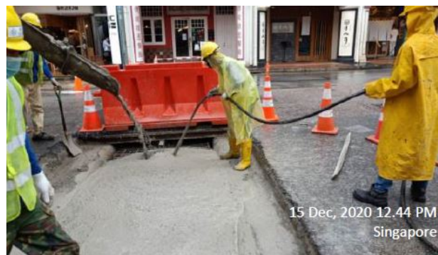
Figure 11: Pouring the cement onto the B10 mesh and pipes
