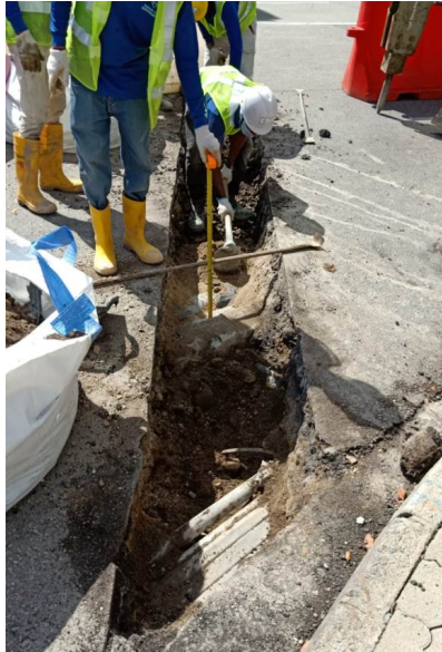
Figure 5: Manual Excavation to avoid damaging any existing cables or pipes.
