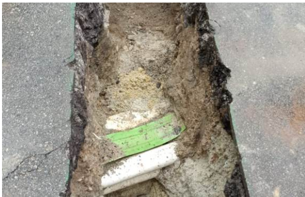
Figure 6: Existing Pipes that were discovered when digging the trial trenches.
