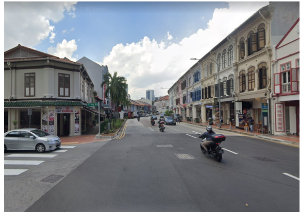
Figure 27: Steel pipes installed along Craig rd - Tanjong Pagar rd junction
