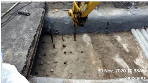
Figure 9: Bakau piling
