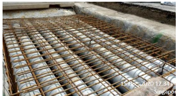
Figure 10: Laying 2 layers of B10 mesh on the steel pipes
