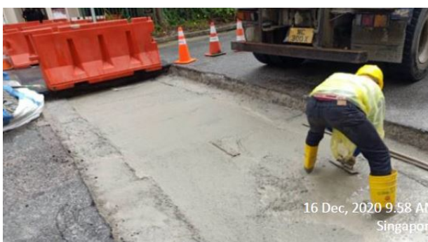
Figure 12: Floating the concrete before applying the Tack coat
