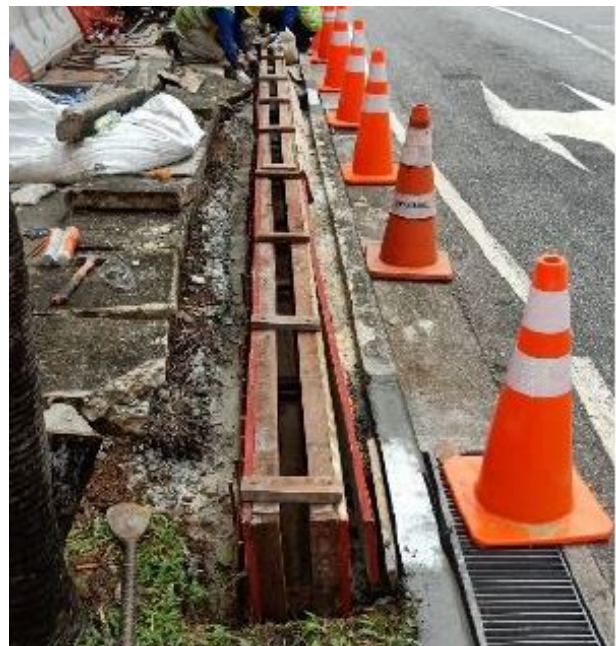
Figure 22: Formwork for type 3 drainage
