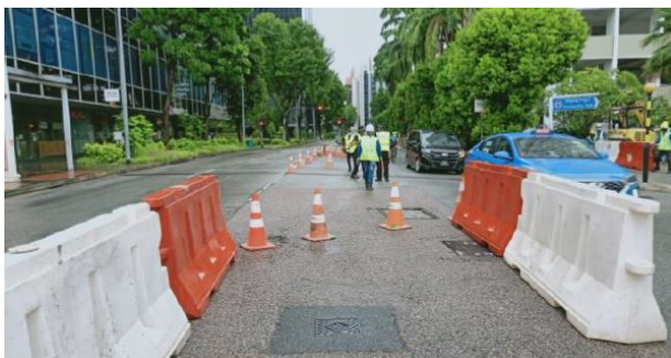
Figure 3: Setting up safety road measures before commencing work
