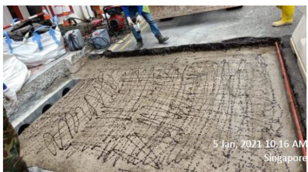
Figure 13: Applying Tack coat on the cement
