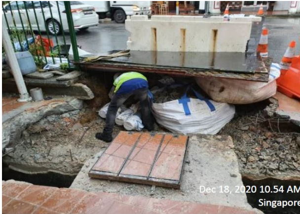
Figure 20: Connecting the Steel pipes to the drainage
