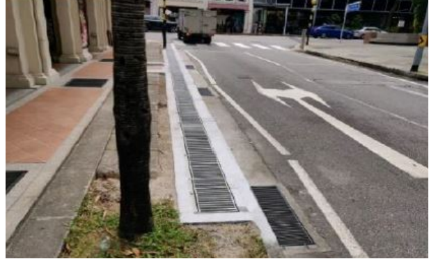
Figure 26: Type 3 drainage completed
